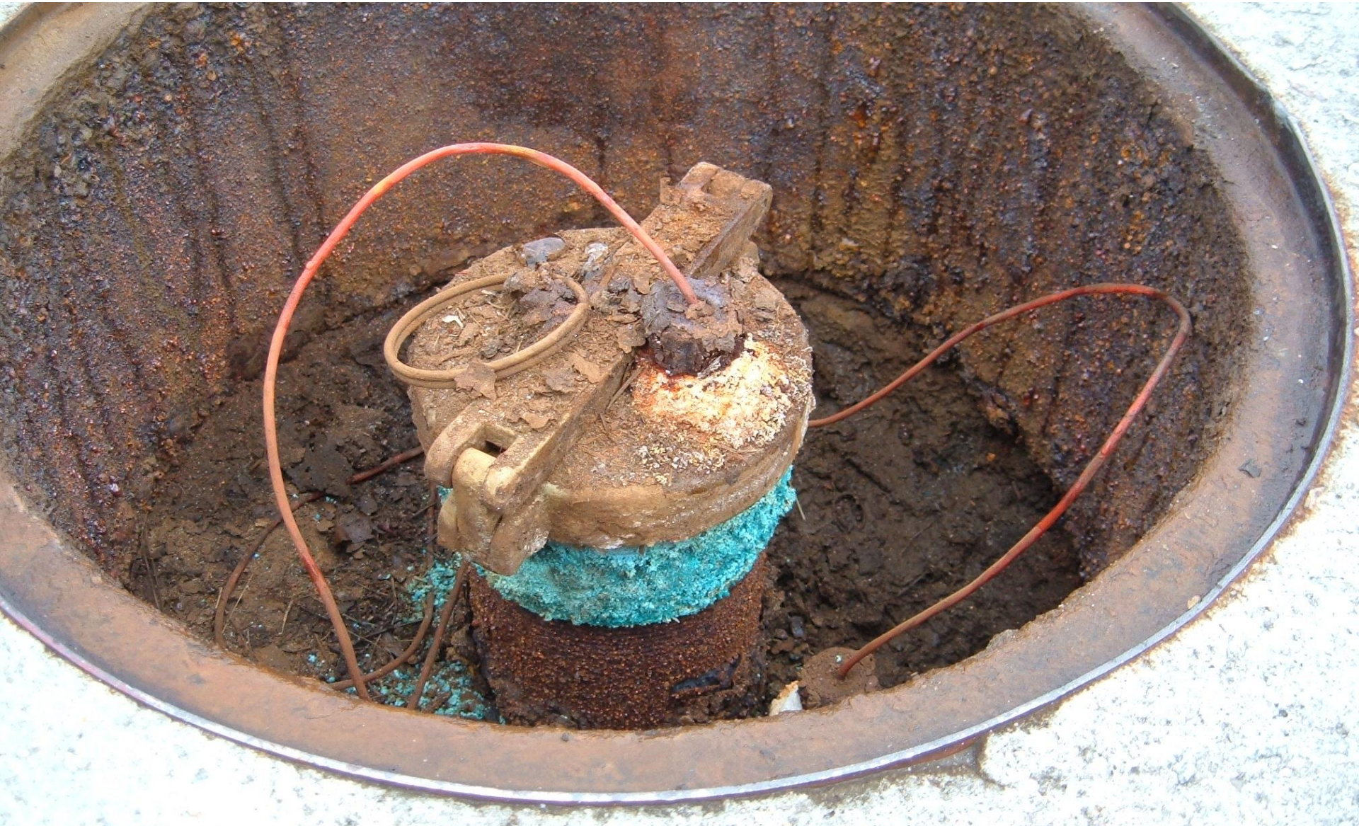
Evidence of vapor leaks
